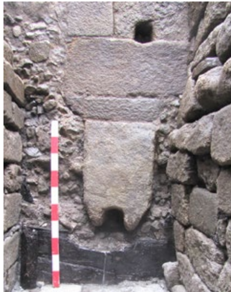
Figure 5: Opus caementicium substratum and wooden formwork visible under the masonry of cloaca 3.
