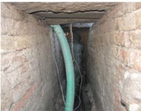
Figure 23: Brickwork in cloaca 2.
