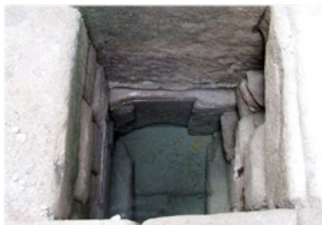
Figure 16: Grooves for sluice gate and conduit into pool A.
