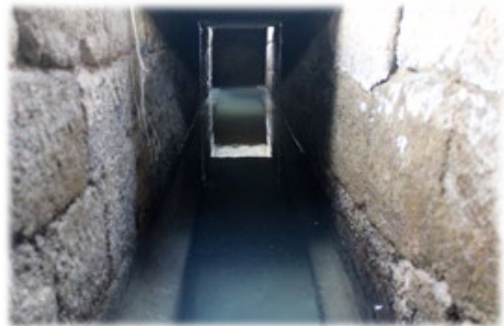
Figure 21: Stone masonry in cloaca 1.
